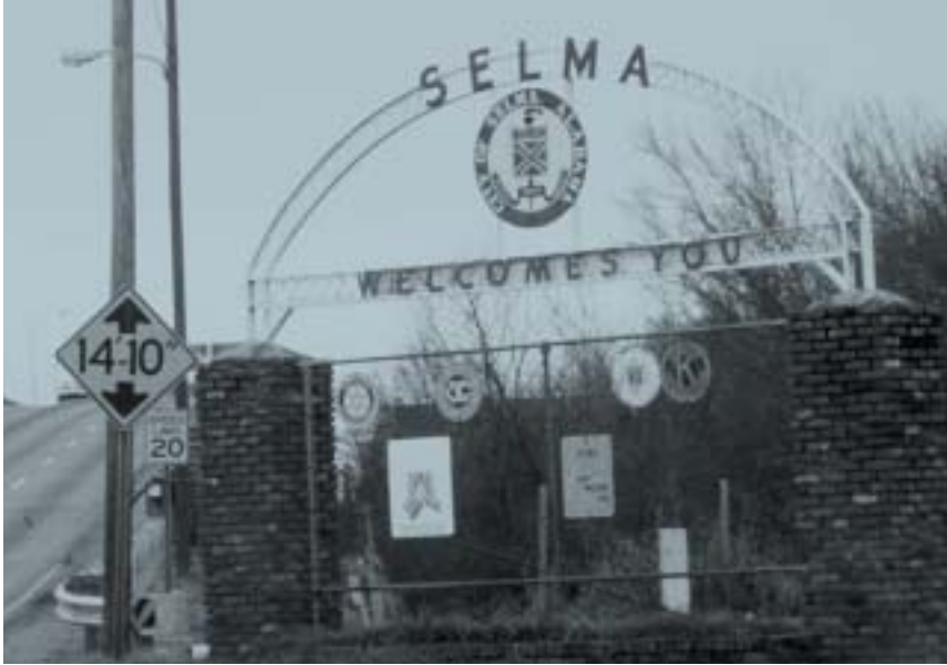
View of proposed project site, Hwy. 80 approaching the Edmund Pettus Bridge. This view shows the site of the "Bloody Sunday" confrontation as it appears today.
